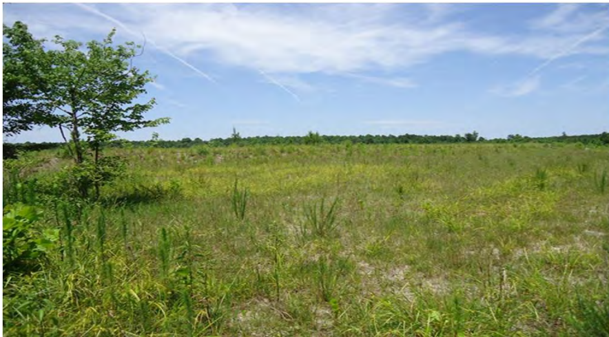
At culvert: NE: Mostly herbaceous veg. on waterline ROW, shrubs, saplings on berm; scattered sweetgum, baccharis south of berm.
